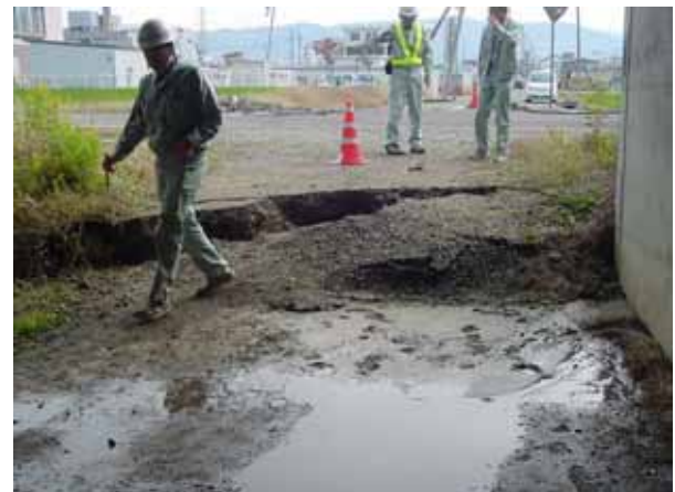
The culvert composed of two sections moved laterally towards the embankment slopes splitting the mid connection and creating opening from which fill soils fell down and partially buried the underpass. The concrete slab sunk about 15-20 cm.
