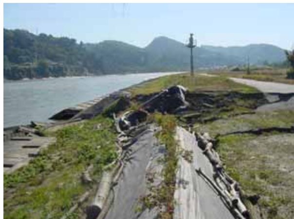
Collapsed portion of the quay wall (Koshino Bridge is seen in the background)
