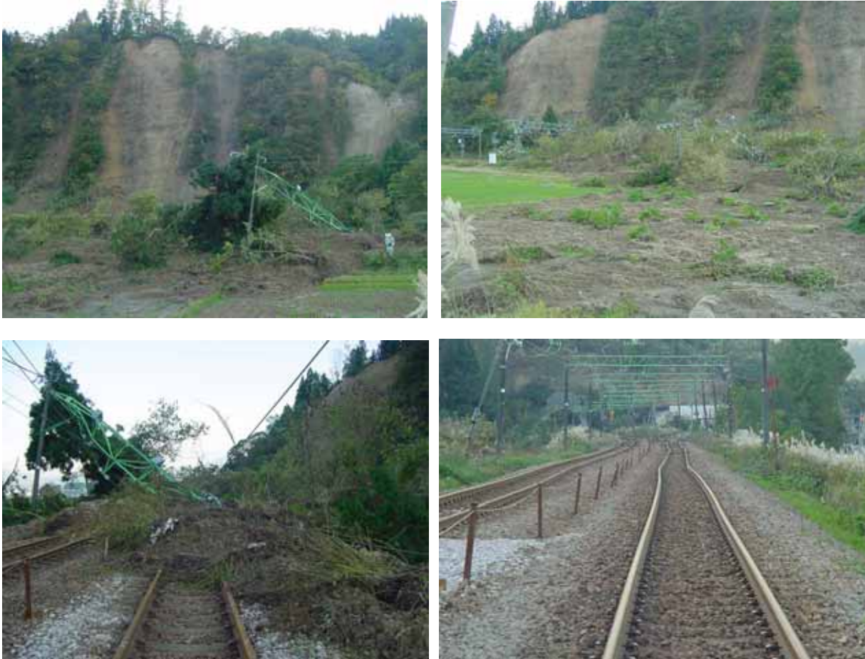
View towards the buried railway (on the left) and in the opposite direction (on the right).
