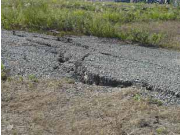
Ground cracks and lateral movement toward the river near the top of the revetment wall.
