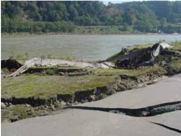
Ground distortion behind the quay wall;
