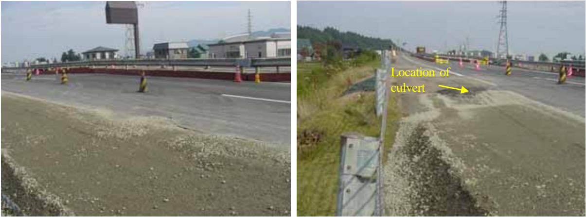
View of the highway from the top of the embankment.
