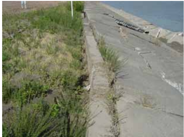
Ground cracks and lateral movement toward the river near the top of the revetment wall.
