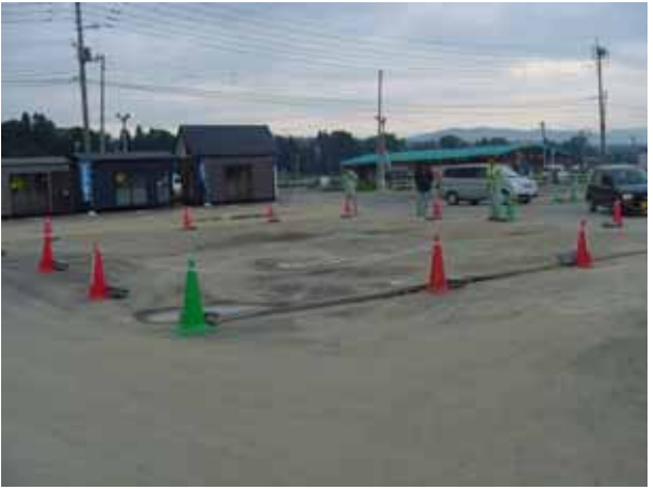
Sand boils and uneven settlement due to liquefaction observed at a parking lot.
