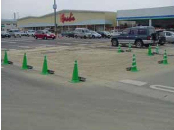
Sand boils and uneven settlement due to liquefaction observed at a parking lot.
