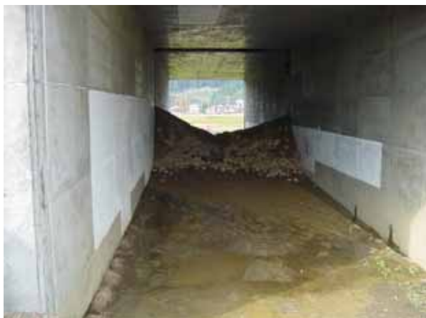
The culvert composed of two sections moved laterally towards the embankment slopes splitting the mid connection and creating opening from which fill soils fell down and partially buried the underpass. The concrete slab sunk about 15-20 cm.
