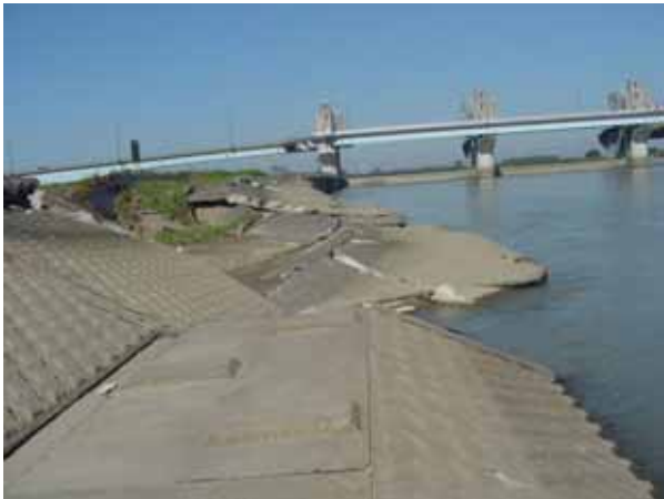
Collapsed portion of the quay wall (Koshino Bridge is seen in the background)
