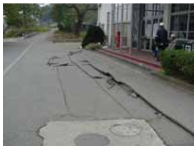
Kawaguchi: Damage in the underground passage of Echigo-Kawaguchi Station (uplift of floor and ground) Location -1
