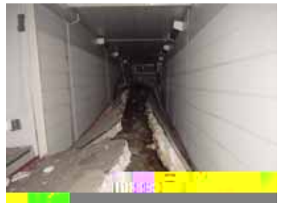
Kawaguchi: Damage in the underground passage of Echigo-Kawaguchi Station (uplift of floor and ground) Location -1
