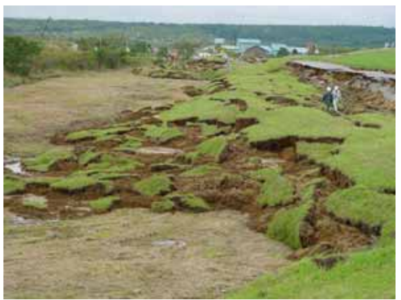
Tokachi River: The largest damage of the embankment occurred near the Ootsu Sewerage Treatment Facility; along two sections with approximate lengths of 150-250 m, the lower body of the embankment completely collapsed; the foundation soil beneath the embankment seen on the left side in the lower images was extremely soft and soaked in water; these images show the first of the two collapsed sections; (C-4)
