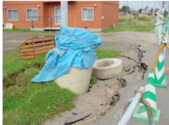
Onbetsu: Additional two man-holes were uplifted as much as 1 m and 1.7 m above the ground level; (B-1)
