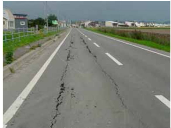
Moiwa: Cracks on asphalt surface and settlement of the road along buried pipelines (D-2)
