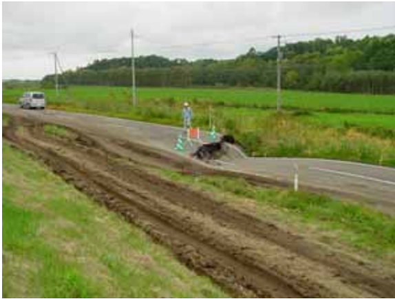
Tabikorai: The road running along the embankment from Moiwa to Ootsu was heavily damaged or collapsed at numerous locations; (C-3)
