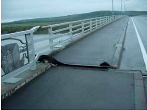
Tokachigawa Bridge: Damage details at the connection of Sections 1 and 2; (C-2)
