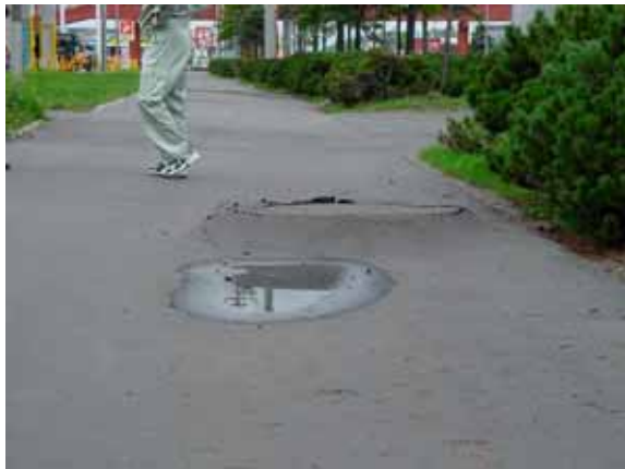
Kushiro: Differential vertical displacement of man-holes on the order of 10-20 cm; part of the movement can be attributed to uplift of the man-hole whereas part is due to settlement of the surrounding ground; the same man-holes were uplifted during the 1993 Kushiro earthquake (A-3)
