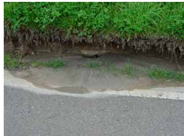
Ootsu: The maximum subsidence was about 40-50 cm; sand boils were seen at the contact zone of the asphalt and ground clearly indicating that the fill soils liquefied; (B-1)
