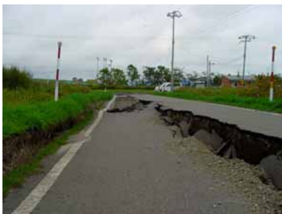
Ootsu: The maximum subsidence was about 40-50 cm; sand boils were seen at the contact zone of the asphalt and ground clearly indicating that the fill soils liquefied; (B-1)
