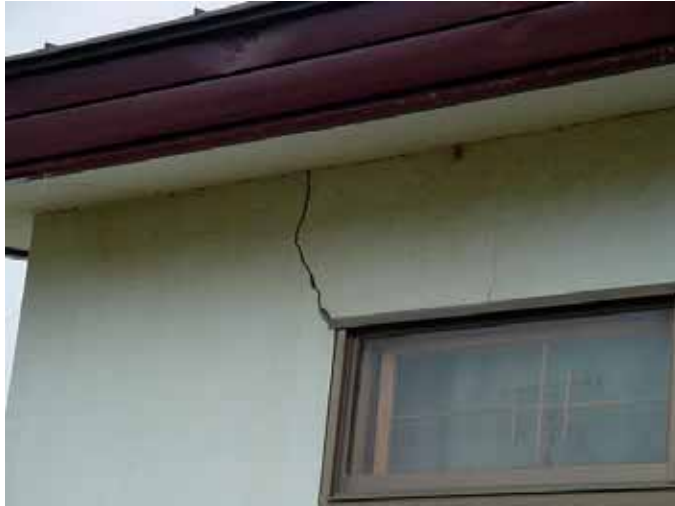
Ootsu: Cracks in the walls and damage due to non-uniform settlements; (south of C-4)
