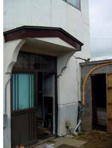
Ootsu: Cracks in the walls and damage due to non-uniform settlements; (south of C-4)
