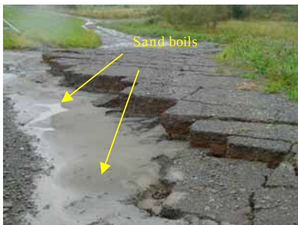
Tokachi River: At this location, massive sand boils were found at the top of the embankment; the approach road shown in the upper-right picture moved laterally; the fissures created by the large lateral movement are seen in-filled with sand-boils and water in the lower images; (C-1)
