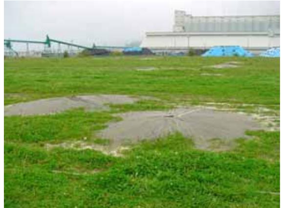
Tokachi Port: Massive sand boils were observed in reclaimed fills; (G-1)
