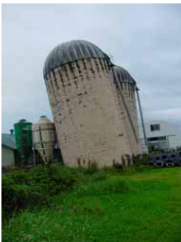
Shinyoshino: Differential settlement and tilting of silo; (C-1)
