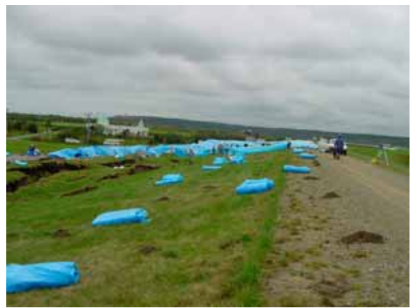
Tokachi River: The second section of the collapsed lower embankment is located just in front of the Ootsu Sewerage Treatment Facility; most of the ground surface was covered with protective sheets and therefore the features of ground distortion were not fully visible; excessive lateral movement of large masses of soil and collapse of the lower body of the embankment were evident; (C-4)
