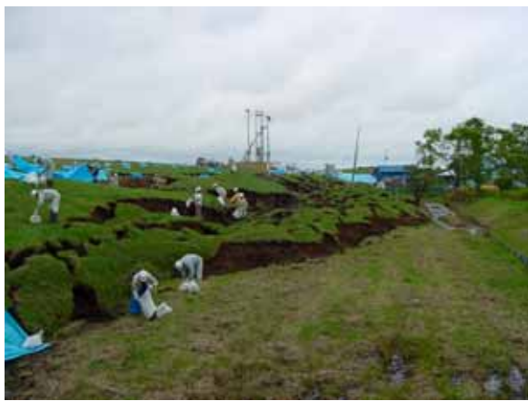
Tokachi River: The second section of the collapsed lower embankment is located just in front of the Ootsu Sewerage Treatment Facility; most of the ground surface was covered with protective sheets and therefore the features of ground distortion were not fully visible; excessive lateral movement of large masses of soil and collapse of the lower body of the embankment were evident; (C-4)
