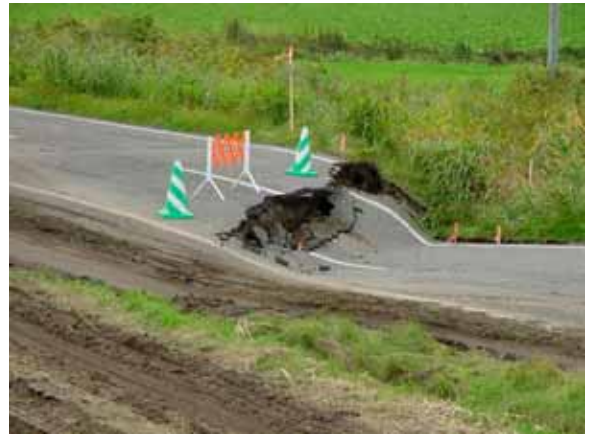
Tabikorai: The road running along the embankment from Moiwa to Ootsu was heavily damaged or collapsed at numerous locations; (C-3)
