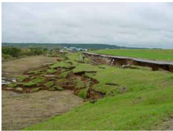
Tokachi River: The largest damage of the embankment occurred near the Ootsu Sewerage Treatment Facility; along two sections with approximate lengths of 150-250 m, the lower body of the embankment completely collapsed; the foundation soil beneath the embankment seen on the left side in the lower images was extremely soft and soaked in water; these images show the first of the two collapsed sections; (C-4)
