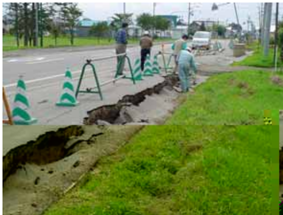
Onbetsu: Collapse of the pavement and subsidence of 30-50 cm was observed along a length of 200-300 m of the pipeline route; the collapsed portion has a width of about 1-1.2 m; (B-1)
