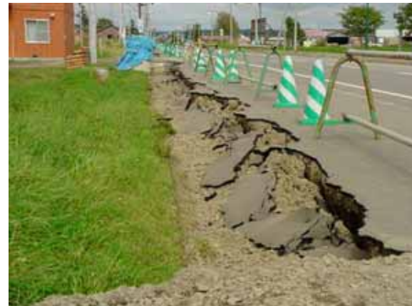
Onbetsu: Collapse of the pavement and subsidence of 30-50 cm was observed along a length of 200-300 m of the pipeline route; the collapsed portion has a width of about 1-1.2 m; (B-1)
