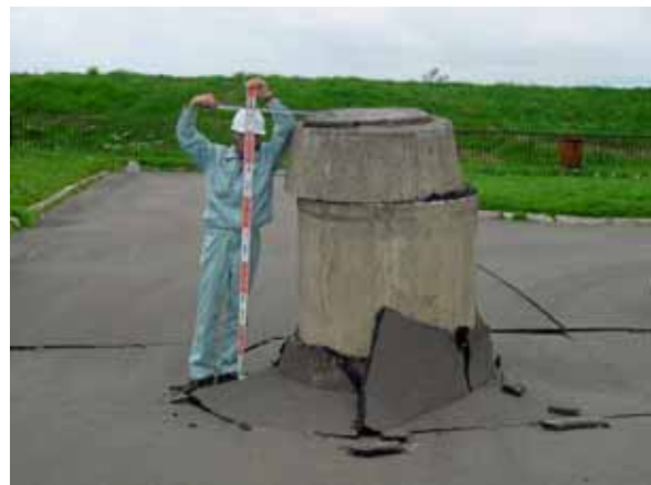
Ootsu: Subsidence of road surface above buried pipelines and uplift of man-holes; the top of the man-hole shown on the right was about 180 cm above the ground level; (B-1)
