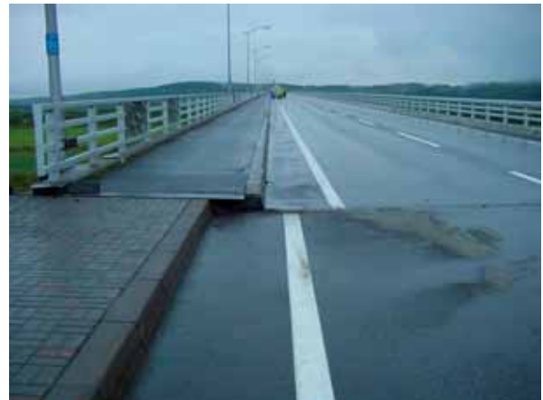
Tokachigawa Bridge: The bridge has two structural systems (Section 1 and Section 2); The upper deck of Section 1 moved laterally towards the right in the picture (NW), about 60 cm, as seen in the image on the left: view from the abutment; (C-2)
