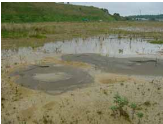
Tokachi Port: Massive sand boils and sand littered on the road surface; (G-1)
