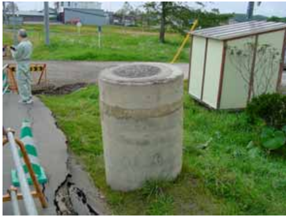
Onbetsu: Huge uplift of a man-hole at Onbetsu, Kawahigashi Danchi; the top of the man-hole was approximately 170 cm above the ground surface; (B-1)
