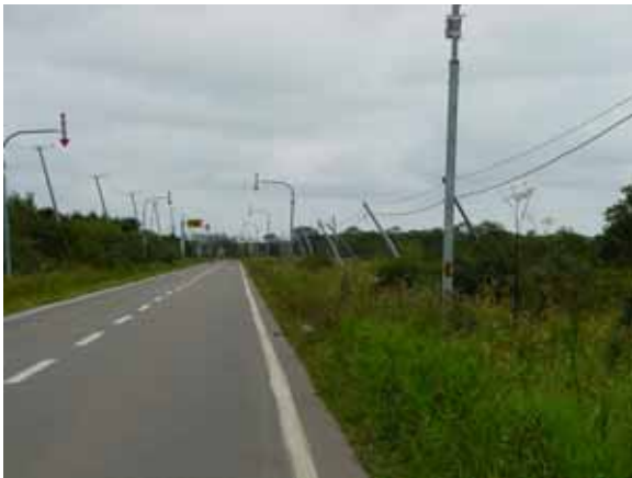
Between Tabikorai and Ootsu: Tilting of distribution poles of electric power lines; sinusoidal wave pattern of tilting was observed with the poles on both sides of the road showing similar pattern of movement; there was no such horizontal wave-pattern in the deformation of the road, which was without damage at this section; (C-3)
