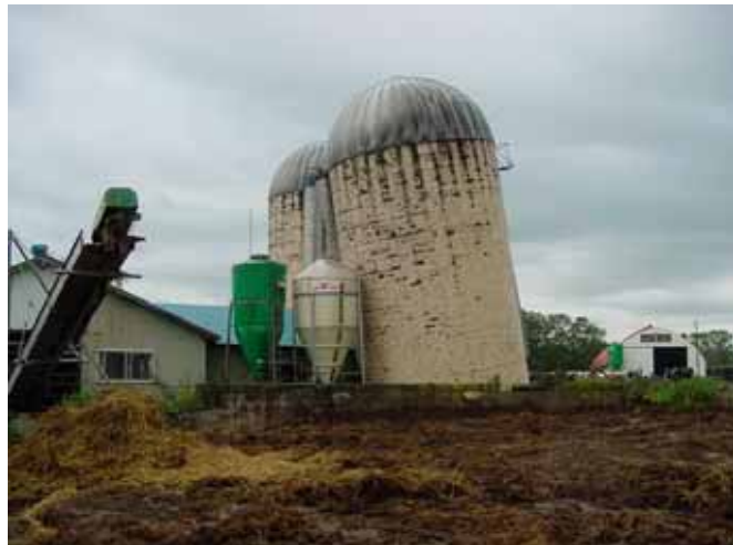
Shinyoshino: Differential settlement and tilting of silo; (C-1)
