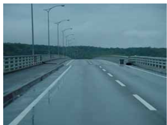
Tokachigawa Bridge: At the connection of two bridge sections: pier at the connection of Sections 1 and 2; View from Section 1 towards Section 2; Section 1 is seen displaced laterally about 60 cm; (C-2)
