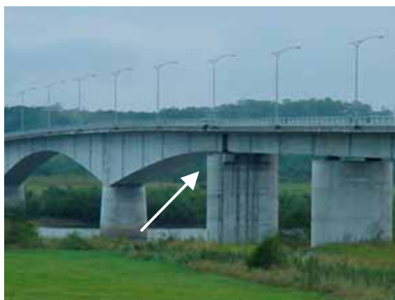
Tokachigawa Bridge: At the connection of two bridge sections: pier at the connection of Sections 1 and 2; View from Section 1 towards Section 2; Section 1 is seen displaced laterally about 60 cm; (C-2)
