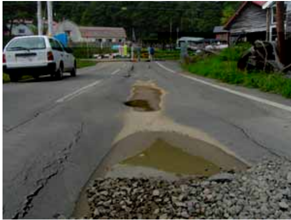
Moiwa: Cracks on asphalt surface and settlement of the road along buried pipelines (D-2)
