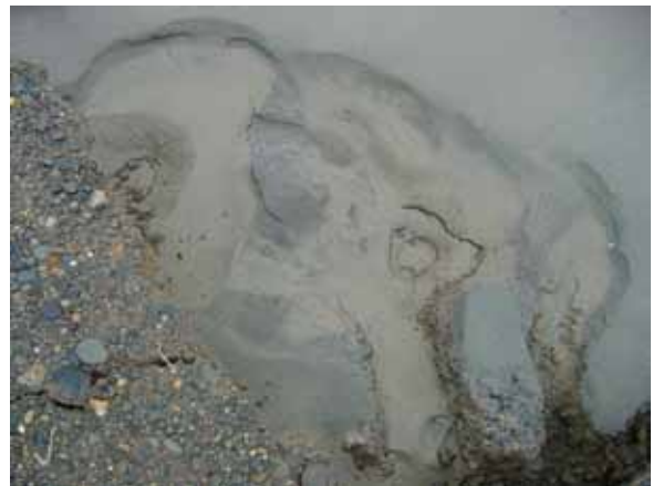
Tokachi River: At this location, massive sand boils were found at the top of the embankment; the approach road shown in the upper-right picture moved laterally; the fissures created by the large lateral movement are seen in-filled with sand-boils and water in the lower images; (C-1)
