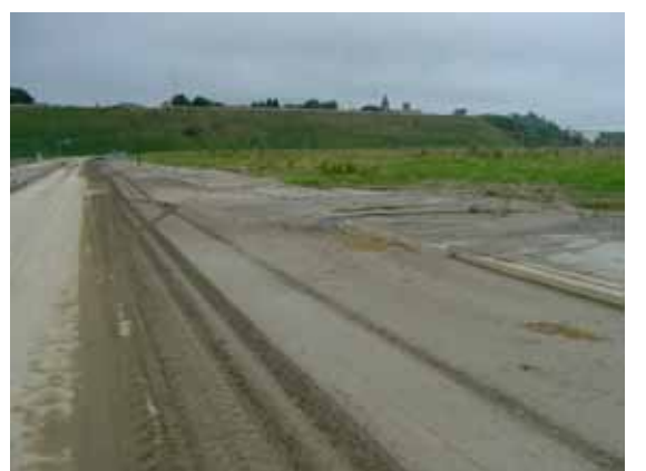
Tokachi Port: Massive sand boils and sand littered on the road surface; (G-1)
