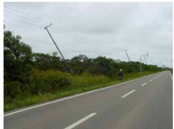
Between Tabikorai and Ootsu: Tilting of distribution poles of electric power lines; sinusoidal wave pattern of tilting was observed with the poles on both sides of the road showing similar pattern of movement; there was no such horizontal wave-pattern in the deformation of the road, which was without damage at this section; (C-3)
