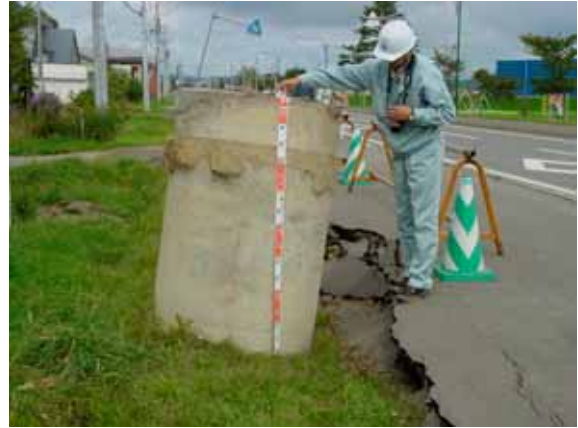
Onbetsu: Huge uplift of a man-hole at Onbetsu, Kawahigashi Danchi; the top of the man-hole was approximately 170 cm above the ground surface; (B-1)
