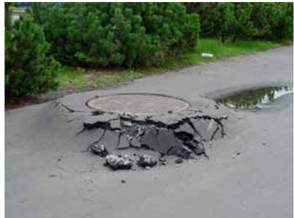
Kushiro: Differential vertical displacement of man-holes on the order of 10-20 cm; part of the movement can be attributed to uplift of the man-hole whereas part is due to settlement of the surrounding ground; the same man-holes were uplifted during the 1993 Kushiro earthquake (A-3)
