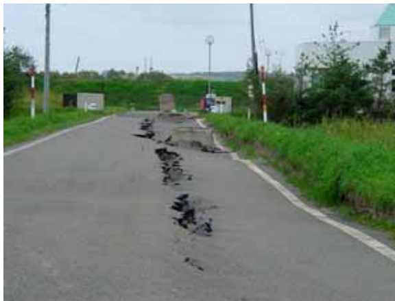
Ootsu: Subsidence of road surface above buried pipelines and uplift of man-holes; the top of the man-hole shown on the right was about 180 cm above the ground level; (B-1)
