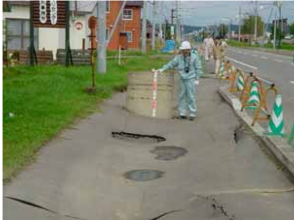
Onbetsu: Additional two man-holes were uplifted as much as 1 m and 1.7 m above the ground level; (B-1)
