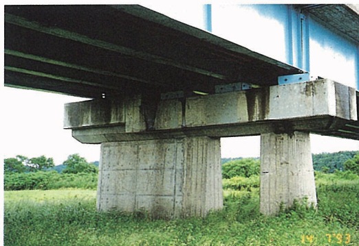
写真4-22 真栄橋の橋脚 Pier of the Shinei bridge
