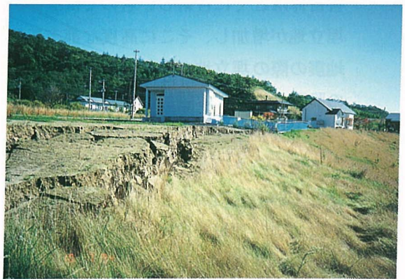
写真－9.10 標茶町茅沼別荘地の盛土被害の比較 Comparison between embankment damage in Kayanuma, Shibecha Town
