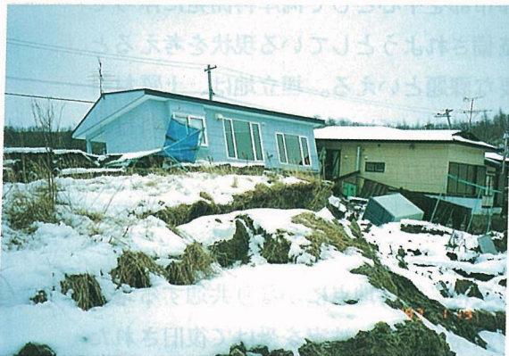
写真－9.10 標茶町茅沼別荘地の盛土被害の比較 Comparison between embankment damage in Kayanuma, Shibecha Town
