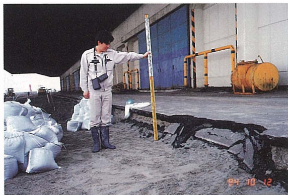
写真-9.3 釧路東港漁業埠頭南側岸壁の段差の比較 Comparison between apron settlement in Fisherman's Wharf, East Port
