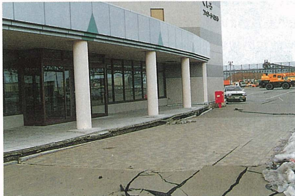
写真-9.4 釧路西港第一埠頭フェリーターミナル駐車場における沈下量の比較 Comparison between the magnitude of settlement in the parking lot of Ferry Terminal
