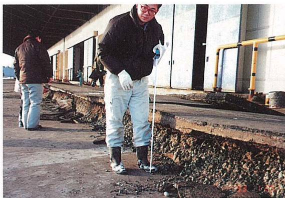
写真-9.3 釧路東港漁業埠頭南側岸壁の段差の比較 Comparison between apron settlement in Fisherman's Wharf, East Port
