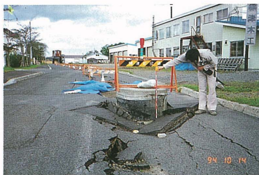
写真-6.7 標津町下水道マンホールの浮き上がりと路面の沈下・陥没 Uplifted manhole and road subsidence in Shibetsu Town
