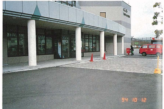
写真-9.4 釧路西港第一埠頭フェリーターミナル駐車場における沈下量の比較 Comparison between the magnitude of settlement in the parking lot of Ferry Terminal
