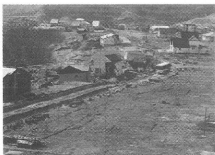
写真9.12 造成地被害の全景 (Photo 9.12 General View of Damaged Site)
