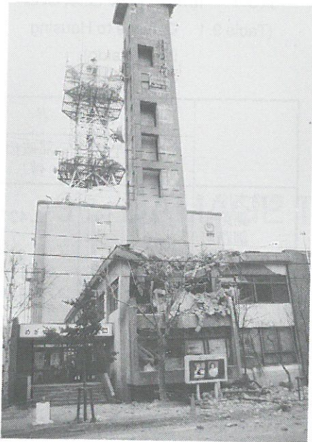
写真9.1 釧路消防署の望楼の被害 (Photo 9.1 Damage to the Watchtower of the Kushiro Fire Station)
