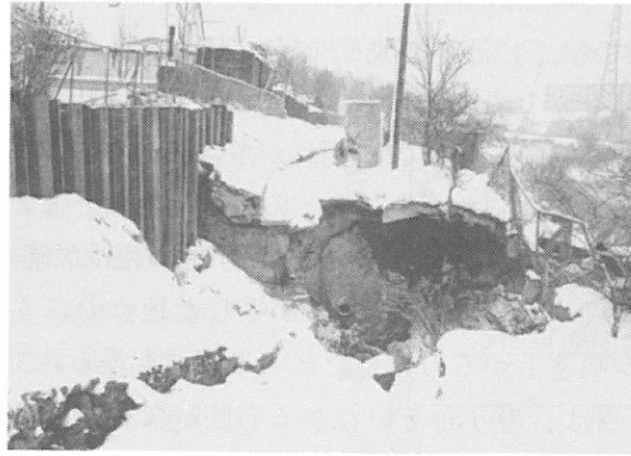
写真9.10 釧路市武佐4丁目27番地わかさ保育園前の斜面崩壊 (Photo 9.10 Slope Failure at 27, Musa 4-chome, Kushiro City)
