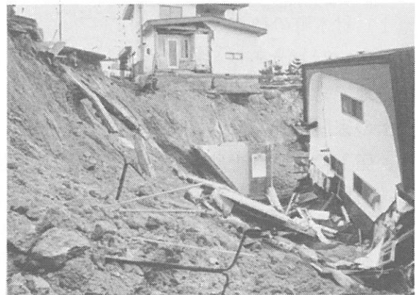
写真9.9 釧路市緑ヶ岡6丁目12番地の斜面崩壊 (Photo 9.9 Slope Failure at 12, Midorigaoka 6-chome, Kushiro City)
