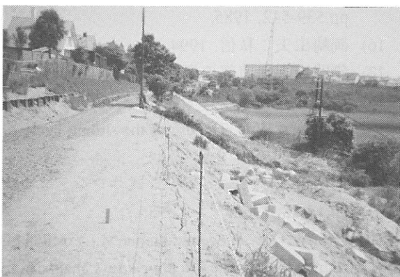
写真9.19 武佐のわかくさ保育園の復旧状況 (Photo 9.19 Repair Work of the Slope of the Wakakusa Kindergarten in Musa)
