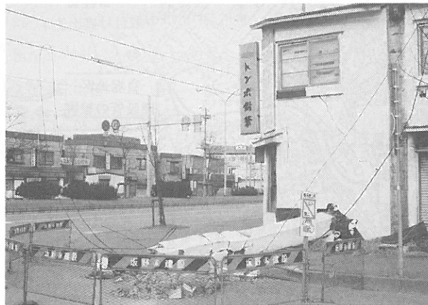
写真9.6 若松町の煙突の崩壊にともなう被害 (Photo 9.6 Damage to a House due to Collapse of Chimney in Wakamatsu-cho)
