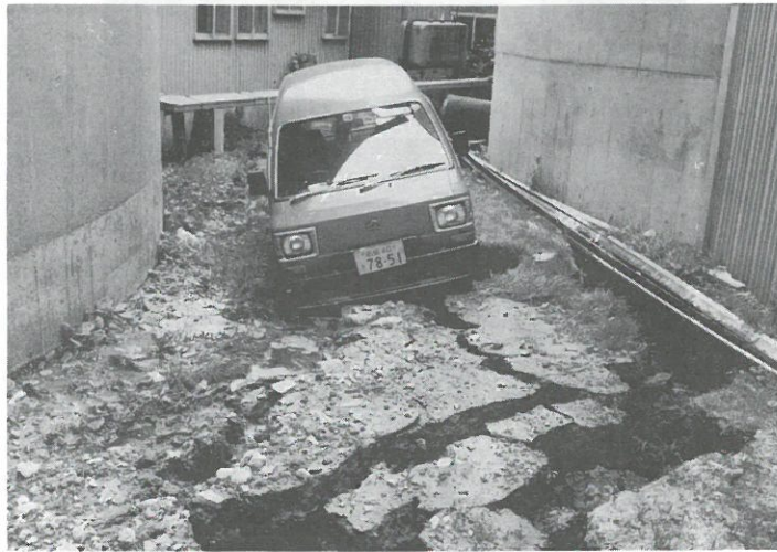
写真10.7 2つのサイロの間には幅1m長さ7mの亀裂 (Photo 10.7 Fissures with 1m Width and 7m Length between the Two Silos)
