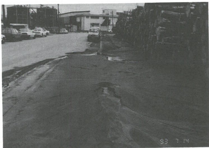
写真10.5 サイロ前面の道路の液状化による噴砂・噴水 (Photo 10.5 Erupted Silty Sand and Water due to Liquefaction along the road in front of the Silo)
