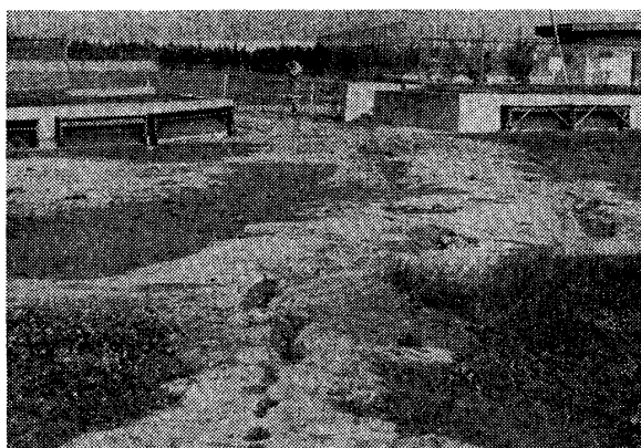
Photo. 9. Boiled sand from fissures in an athletic field (Site A-6)
