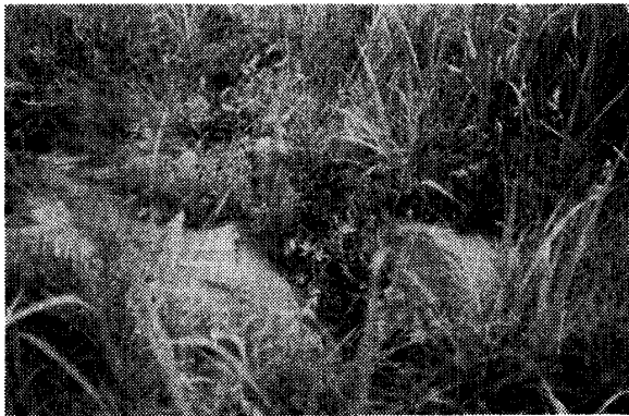
Photo. 7. Boiled sand at outside base of dike along the Yoshida River (Site Q-1)
