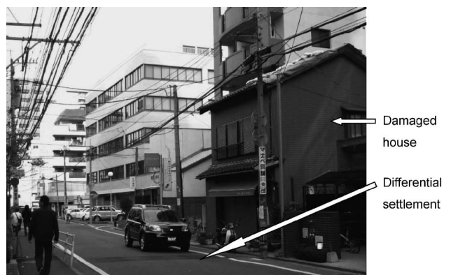
Photo 9 Differential settlement observed above the Kego Fault
