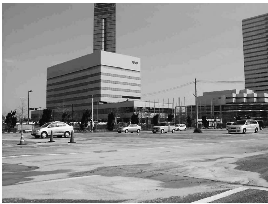
Photo 4 Boiled sand in Momochi-hama
