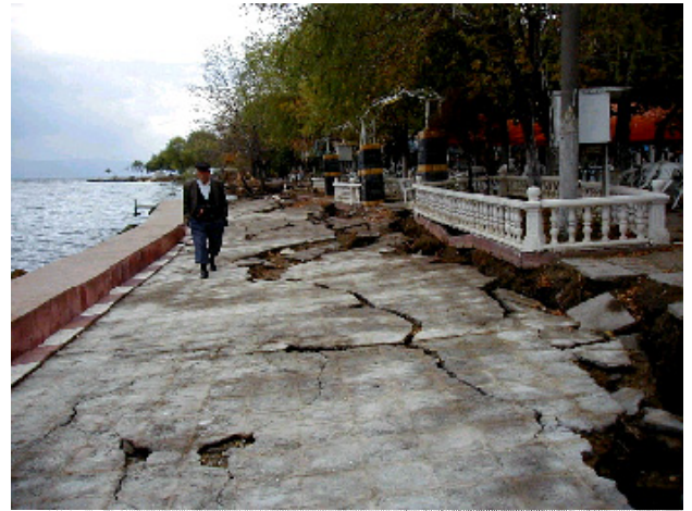
Photo. 6. Subsidence of the ground with cracks parallel to the shoreline
