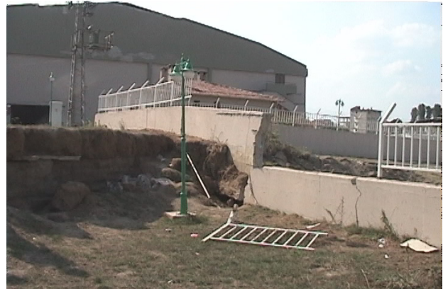
Photo. 16. Vertical dislocation of a branch fault
