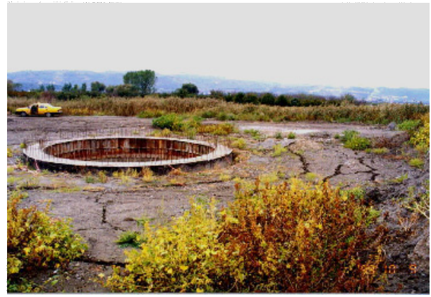
Photo. 3. Cracks near the circular diaphragm wall
