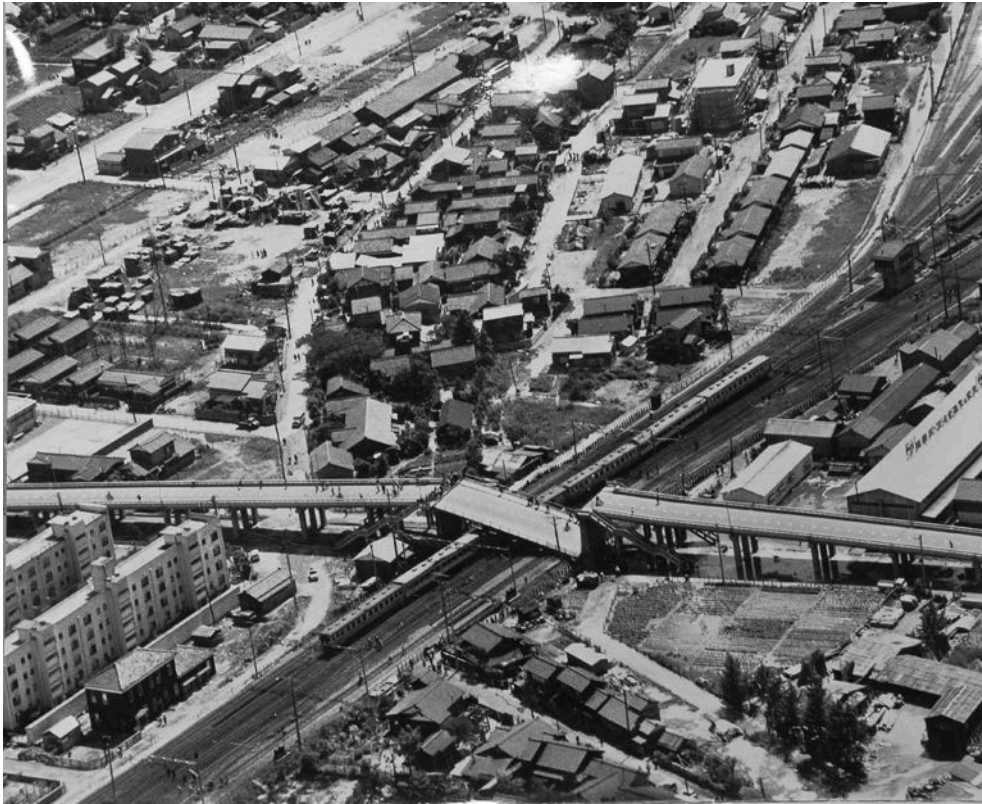
Fig. 46. Damage of railway overpass bridge (1) (still photo taken by Mr. Yuminamochi) 東跨線橋の落下(1)
