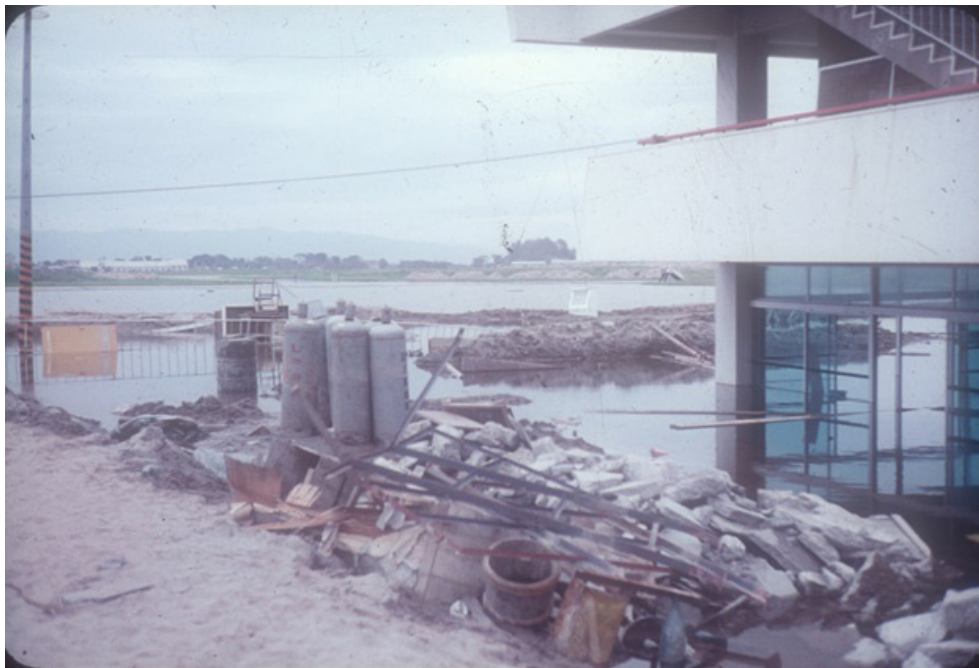
Fig. 55. 1.2-meter subsidence of airport building caused by liquefaction (no damage in structure and window glasses) (University of Tokyo) 後日撮影した空港ビルの沈下状況
