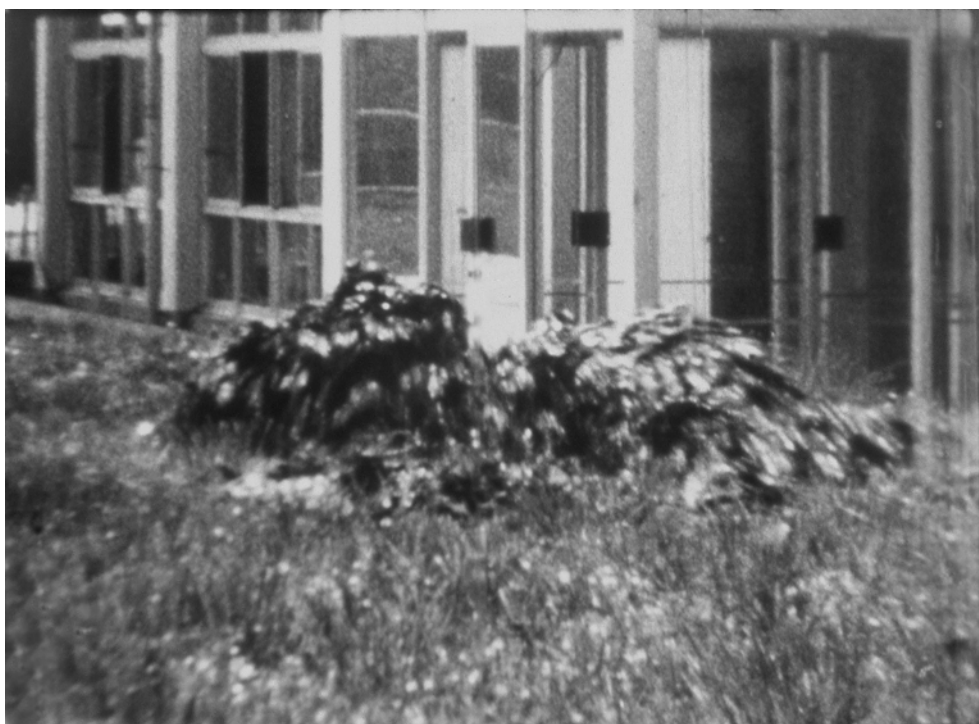
Fig. 7. Beginning of ejection of sand and water in front of the terminal building (captured from Mr. Yuminamochi's motion picture) 噴砂噴水の始まり
