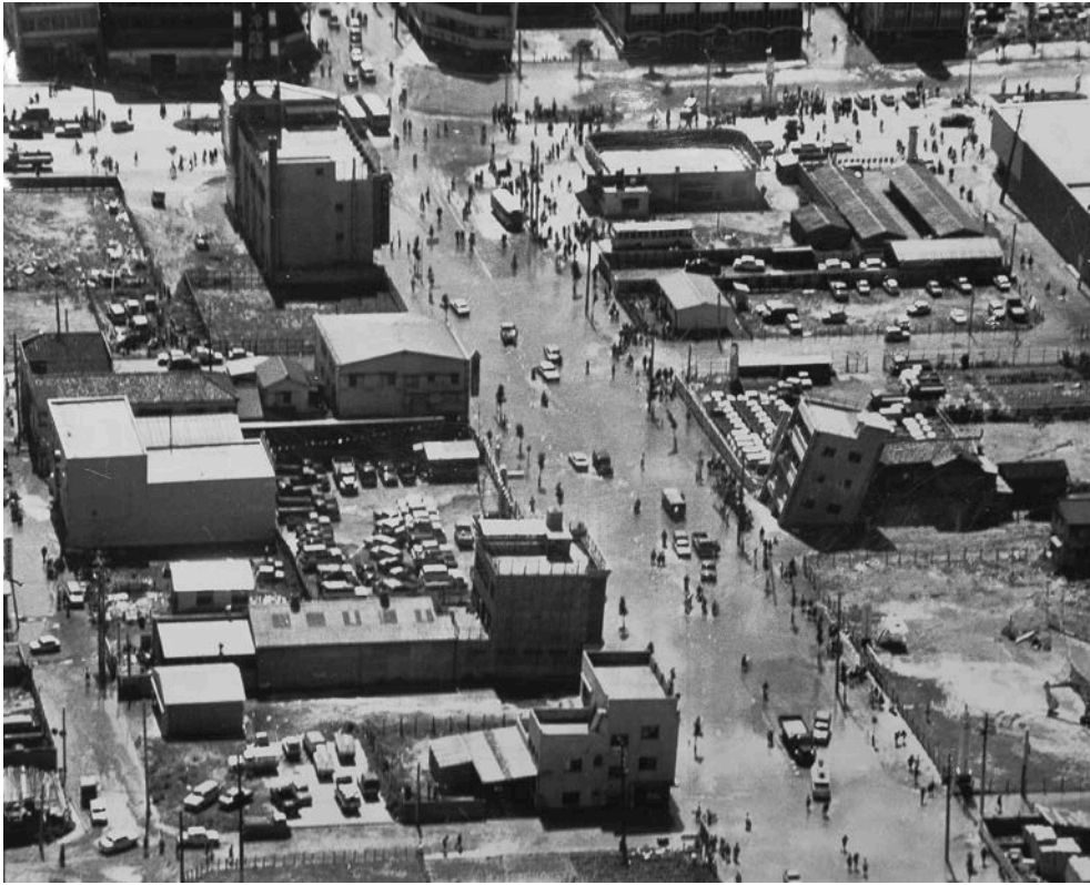
Fig. 40. Akashi Street near the Niigata Station in which the road surface is flooded by liquefaction ejecta 明石通りの液状化被害
