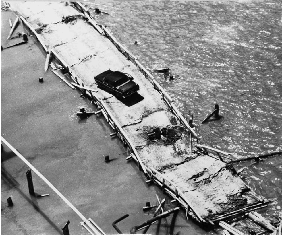
Fig. 50. Fall-down of Matsuhama Bridge across the Agano River (a new bridge was under construction next to this old one at the time of the earthquake) (still photo taken by Mr. Yuminamochi) 阿賀野川に架かる松浜橋（旧橋）の落橋
