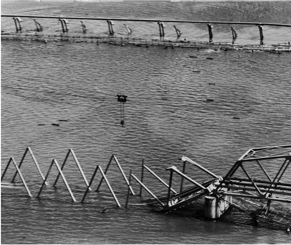
Fig. 52. Collapse of both old and new Matsuhama Bridge (the new bridge in front was under construction) (still photo taken by Mr. Yuminamochi) 工事中の松浜橋新橋も1スパン落橋
