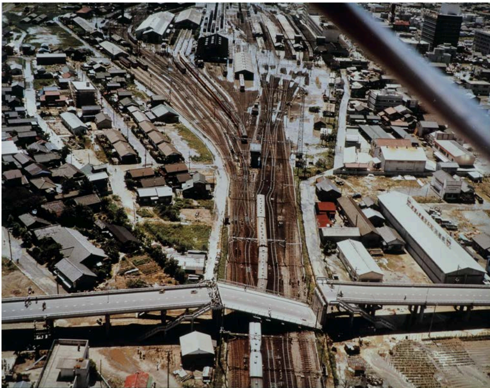
Fig. 47. Damage of railway overpass bridge (2) (still photo taken by Mr. Yuminamochi) 東跨線橋の落下(2)
