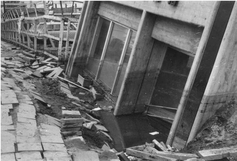
Fig. 43. Damage detail of the tilted building in Figs. 41 and 42 (Reconnaissance team of Civil Engineering Department, University of Tokyo) ビルディングの傾斜状況の詳細
