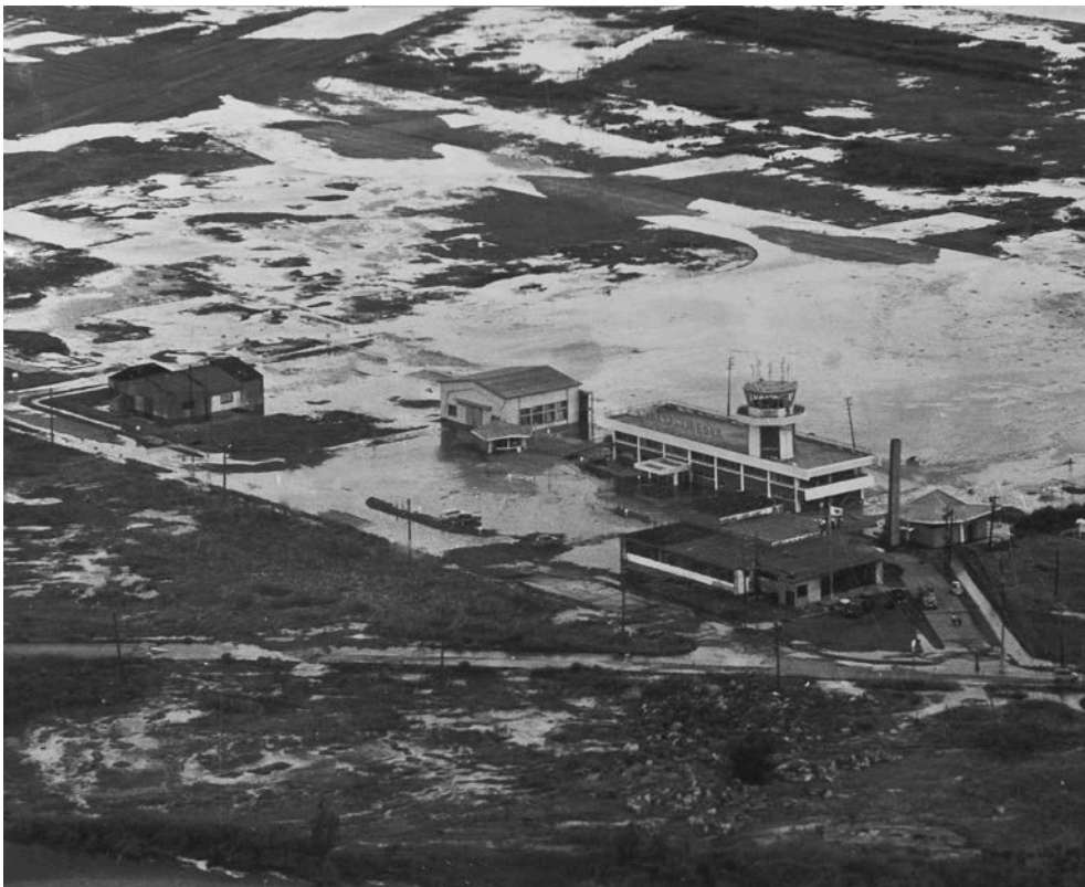
Fig. 54. No structural damage in the airport building in spite of its substantial liquefaction-induced subsidence (still photo taken by Mr. Yuminamochi) 甚大な液状化に比して構造物に被害の無いことが特徴
