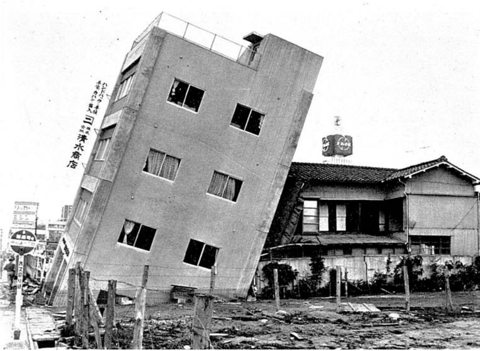
Fig. 42. Contrast in damage extents of heavier RC building and lighter wooden two-storey house 17) (this photograph can be used for academic/engineering purposes freely with reference to the literature 17; no request for permission needed) RC ビルの傾斜と木造家屋の無被害（軽微な変状か）との対比
