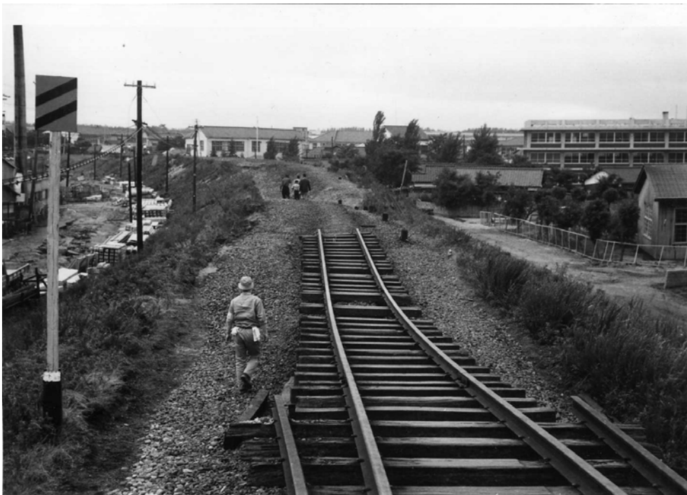
Fig. 38. Subsidence and lateral spread of the Echigo Line railway embankment (Shinano River and Kawagishi-Cho Apartment Buildings located to the left of this picture) (photograph by University of Tokyo) 越後線盛土の変状
