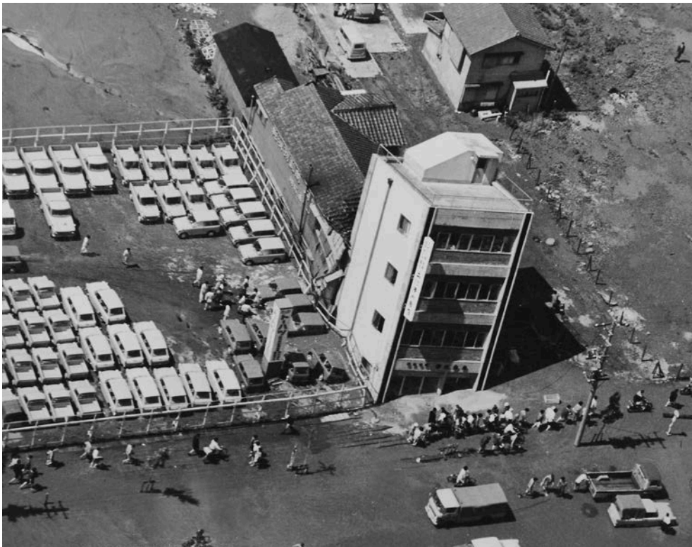
Fig. 41. Tilting of RC building in Akashi Street resting on liquefied subsoil (still photo taken by Mr. Yuminamochi) 傾斜したビルディング
