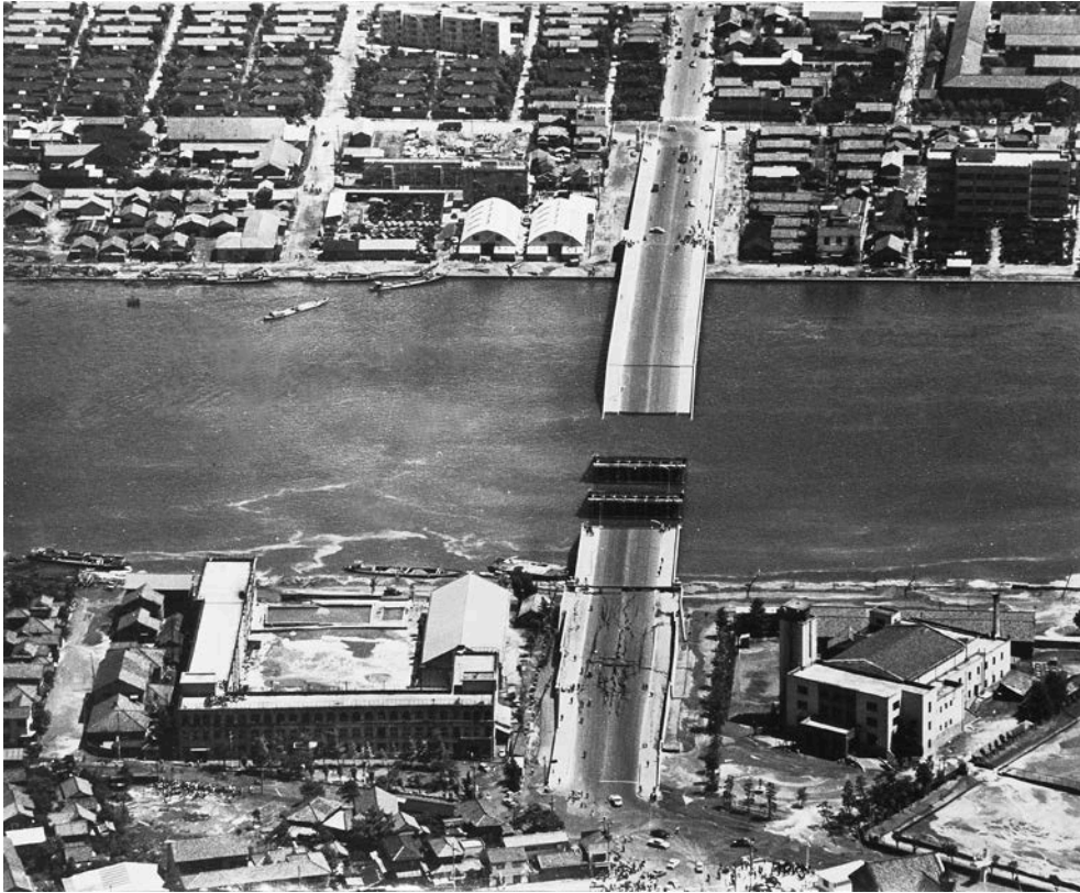
Fig. 28. Fall of Showa Bridge and the substantial damage of the revetment wall along the river (2) (downstream to the left) (still photo taken by Mr. Yuminamochi) 昭和大橋近隣の護岸の被害
