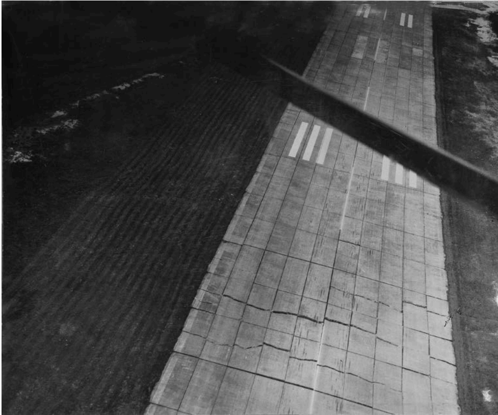
Fig. 57. Cracks and distortion of the airport runway due to heterogeneous subsidence after liquefaction (still photo taken by Mr. Yuminamochi) 滑走路の変状
