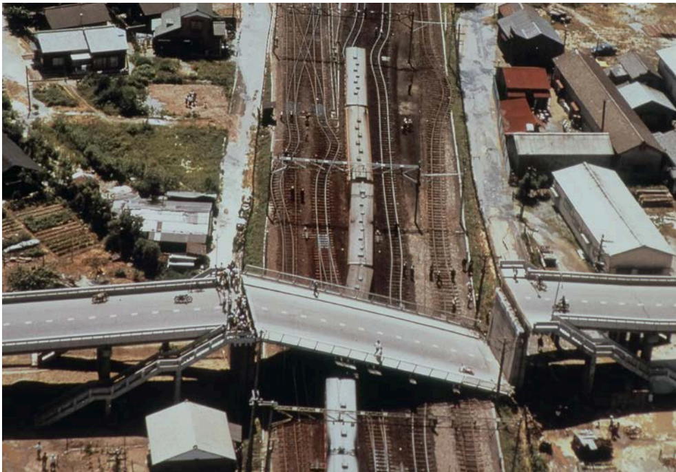
Fig. 49. Damage of railway overpass bridge (4) (still photo taken by Mr. Yuminamochi) 東跨線橋の落下(4)
