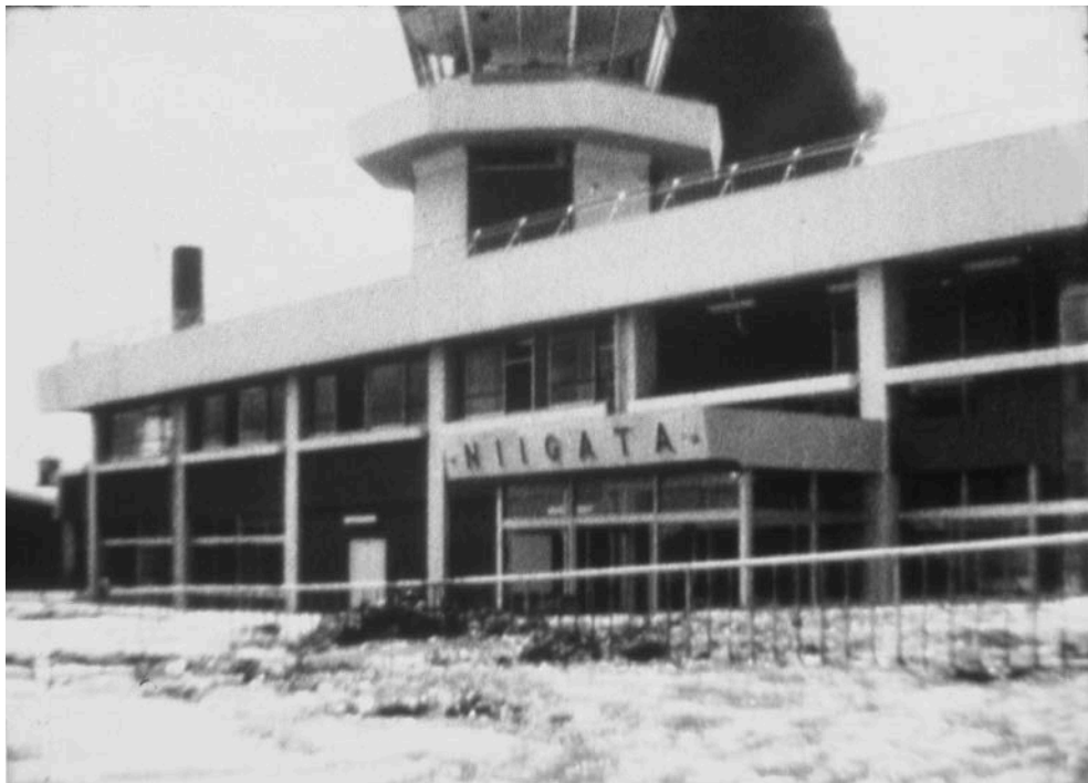
Fig.11. Terminal building inundated by deeper ejected water (captured from Mr. Yuminamochi's motion picture) 水没しつつある空港ビル
