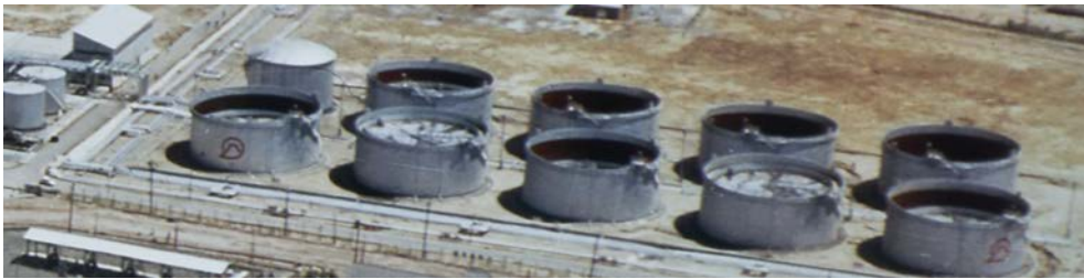
(b) Broken roof of oil tanks (partially enlarged photograph) タンクの被害
