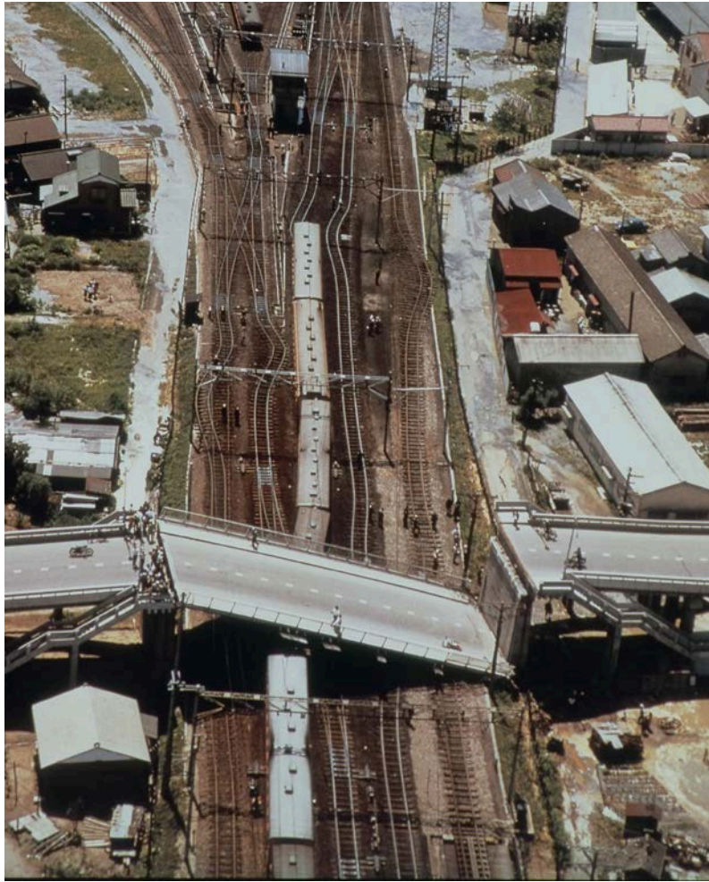
Fig. 48. Damage of railway overpass bridge (3) (still photo taken by Mr. Yuminamochi) 東跨線橋の落下(3)
