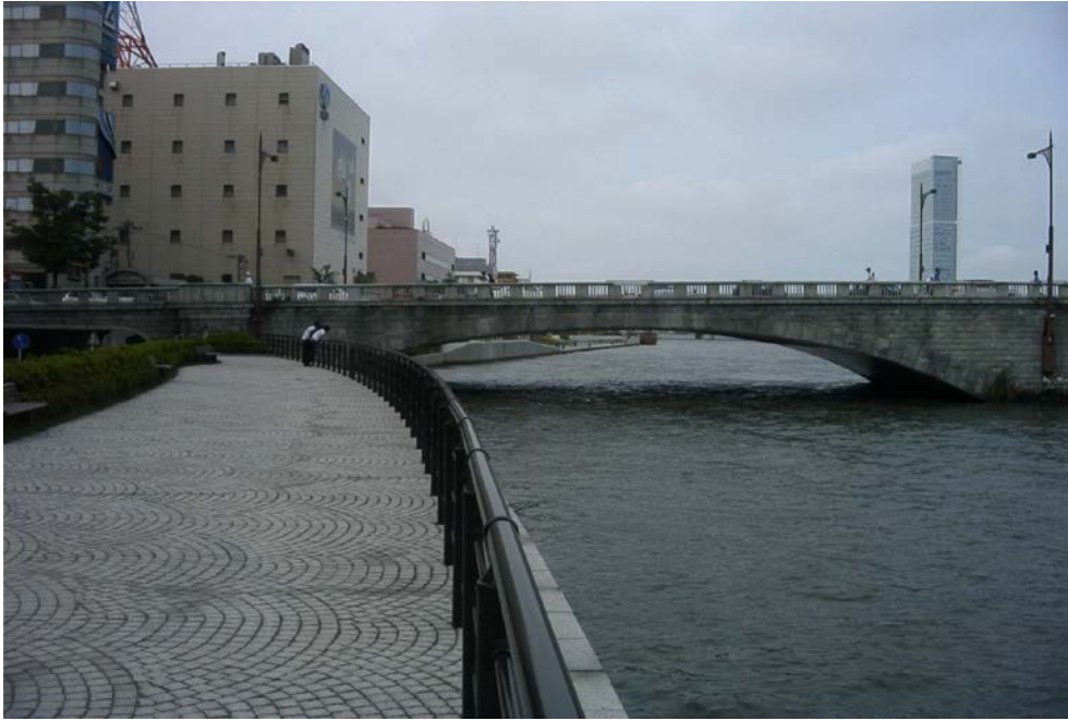
Fig. 26. Distorted shape of the revetment wall in 2003 at the northern side of the Bandai Bridge (IITT Imagery Bank) 万代橋北たもとの護岸の曲線型変状
